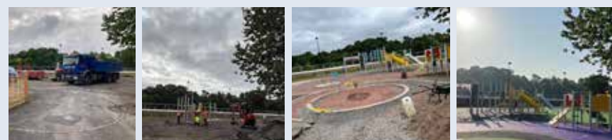
From a building site... To laying strong foundations... To starting to place the equipment... To a modern, child friendly park ready to welcome local families.
